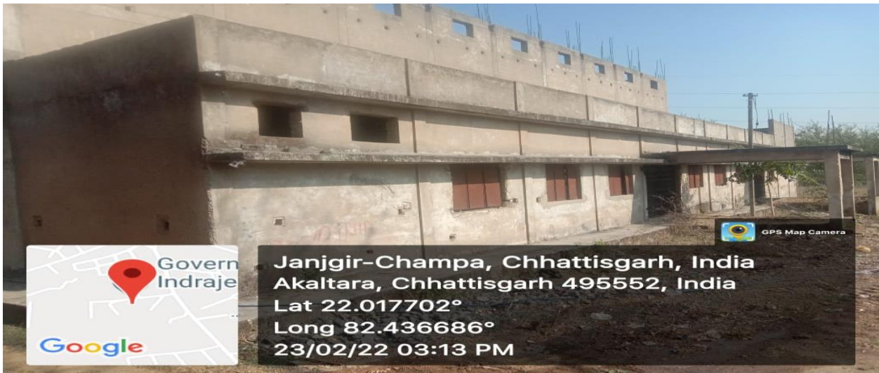
Indoor Stadium (Under Construction)
